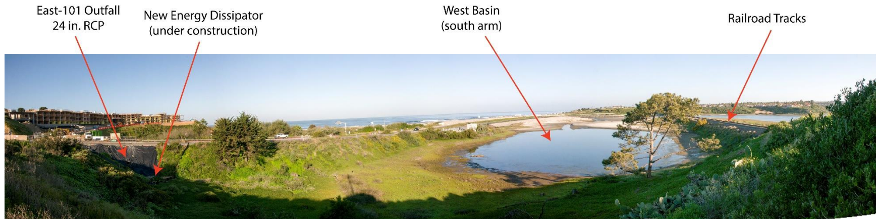
Figure 1: View of major components of the North Coast Highway 101 infrastructure improvements in the south arm of the West Basin of Batiquitos Lagoon including East 101 Outfall enhanced by new energy dissipator,
