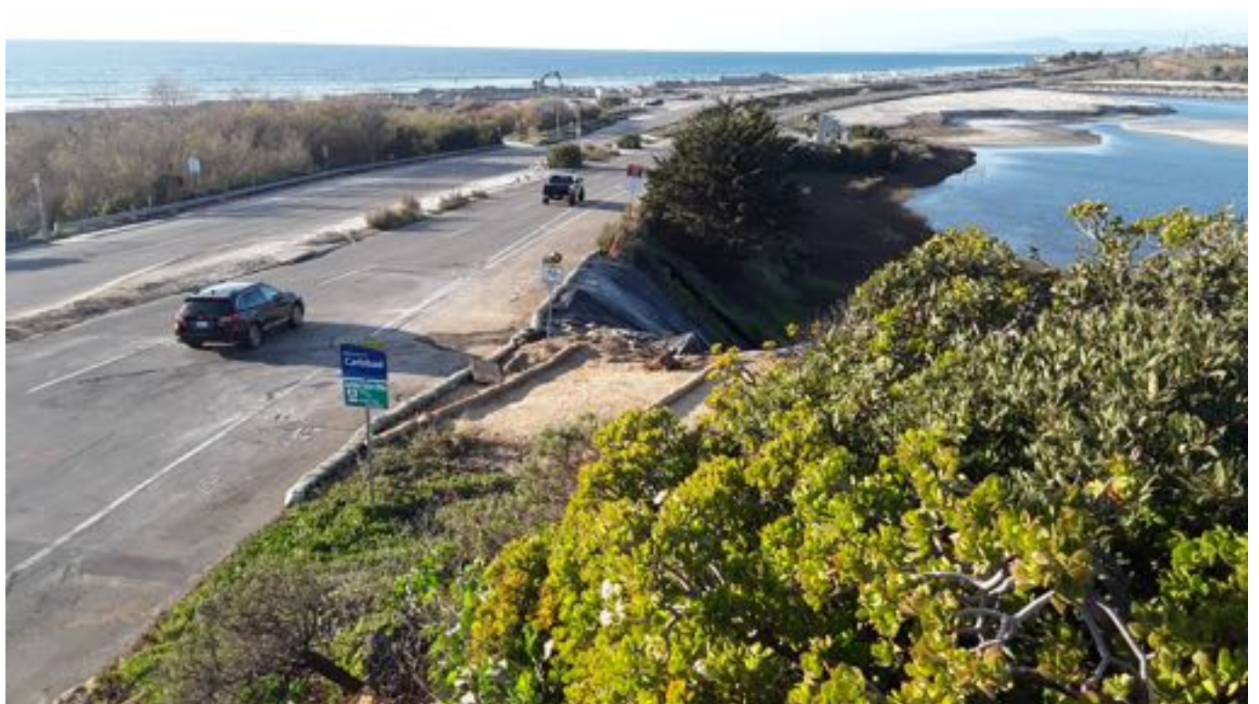
Figure 11: New construction on 2020-01-17 undercover.
