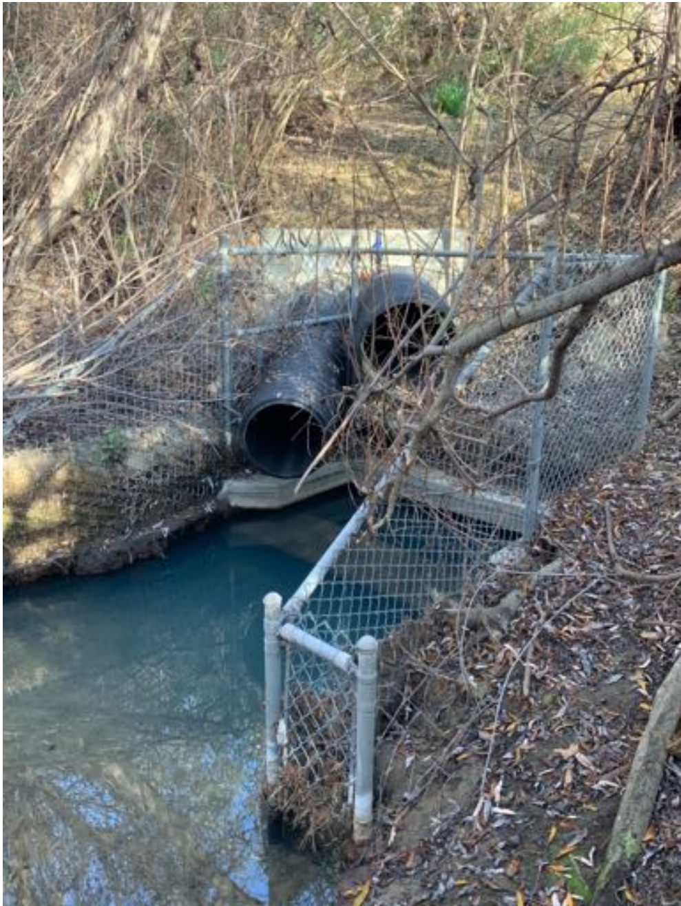
Figure 9: Storm sewer outfall into Batiquitos Lagoon.
