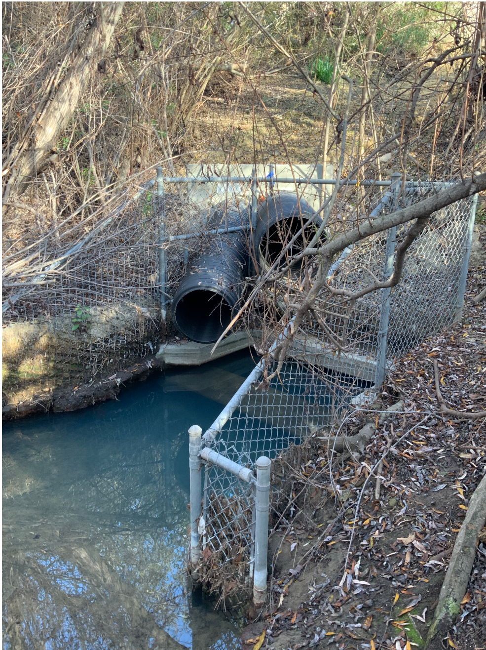
Figure 9: Storm sewer outfall into Batiquitos Lagoon.
