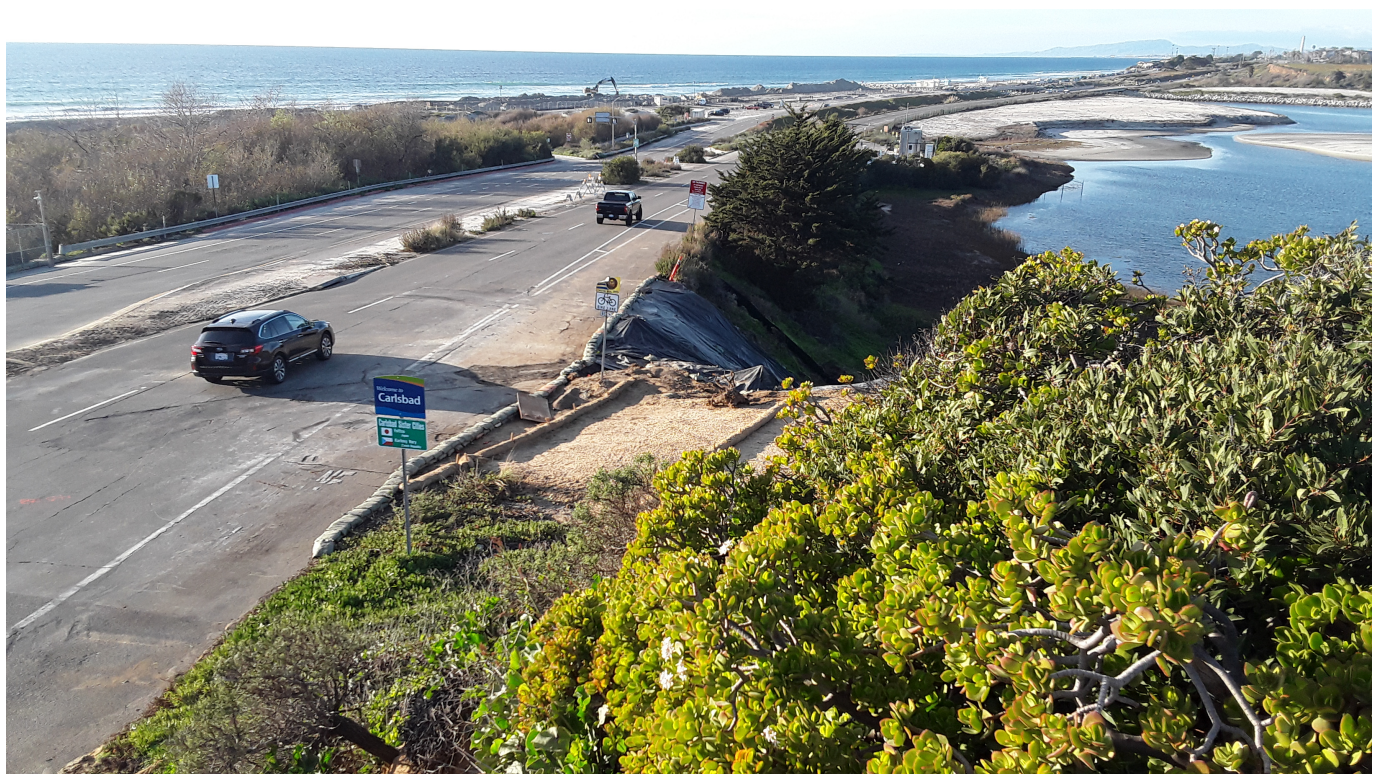
Figure 11: New construction on 2020-01-17 undercover.
