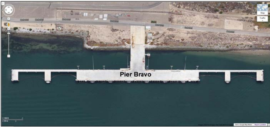
Figure 5-243. Google Earth photo showing the configuration of Ammunition Pier Bravo at NBC (Image: Google).
