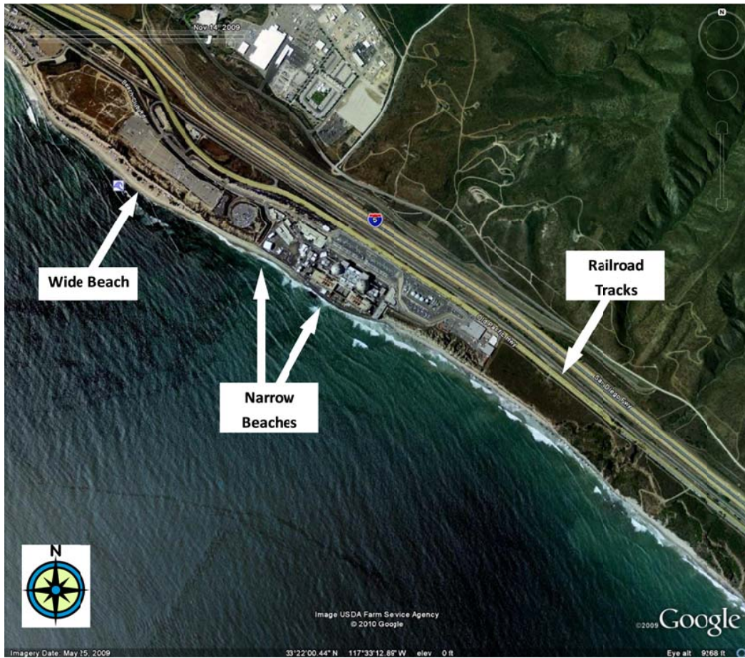
Figure 3-28. Google Earth image taken 25 May 2009 of about 4 km of coast at SONGS shows the greatly reduced beach widths at and adjacent to the power plant (see text). Note the railroad tracks that lie coastward of I5.
