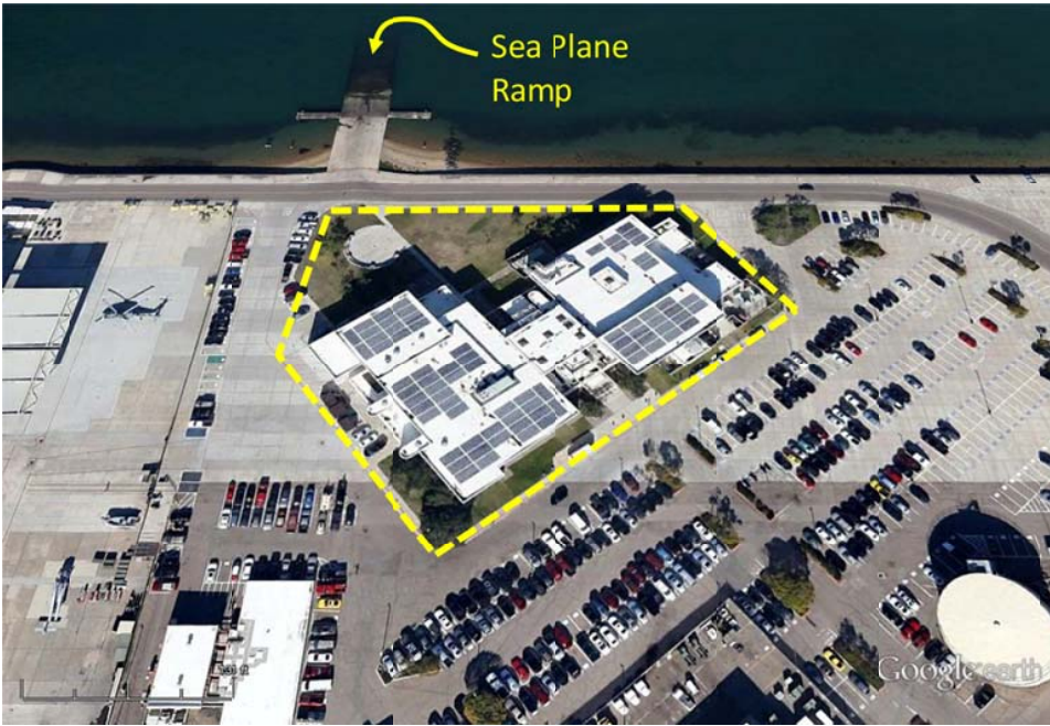
Figure 5-235. Naval Base Coronado looking north at the Helicopter Training Facility. The building is located approximately 70-ft from San Diego Bay.
