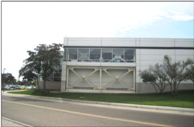
Figure 5-236. Naval Base Coronado with the Helicopter Training Facility as seen from Moffett Road. The exterior surface (lawn) berms up towards the building to lessen the impact of the wall elevation. The interior finish floor is approximately 30-in. below adjacent exterior grade.
