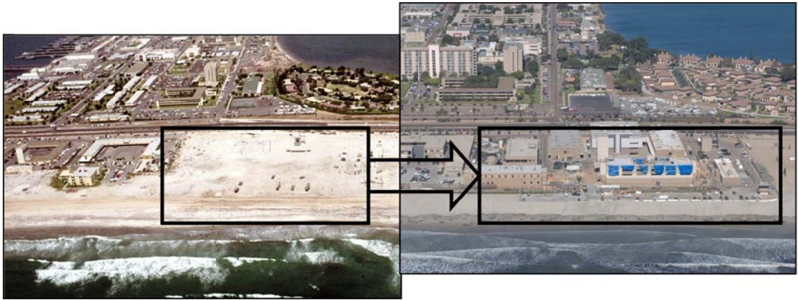
Figure 3-44. (Left) Photo of NAB ocean front facilities taken in 1972 (Cal Boating Image 958012 from CA Coastal Records Project). (Right) Photo of same area taken 19 September 2008 with additional construction on back beach (black boxes) and denser bayside housing (CA Coastal Records Project Image 200805108; Copyright (C) 2002-2014 Kenneth & Gabrielle Adelman, California Coastal Records Project, www.Californiacoastline.org ).
