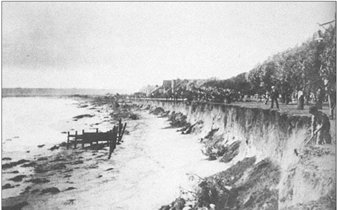
Figure 3-42. View to the northwest from the Hotel Del Coronado after large wave storm from the south caused massive beach erosion in 1905 (Courtesy of the Center for Coastal Studies, Scripps Institution of Oceanography, University of California, San Diego).
