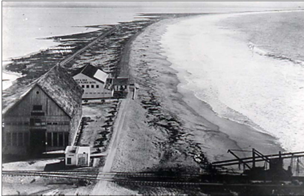
Figure 3-45. Photo taken from the Hotel Del Coronado cupola looking south over Silver Strand in 1898 (Courtesy the U.S. Grant IV collection). Note the narrow ocean beach (right) and over-wash fans on the bayside (left).
