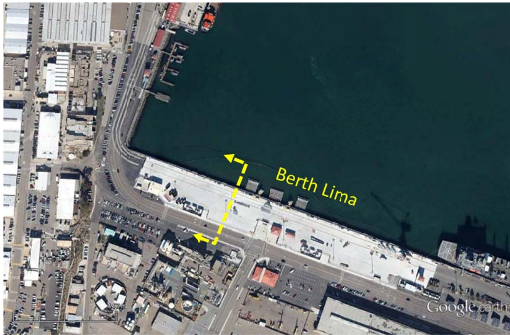
Figure 5-277. Google Earth aerial view showing the configuration of Berth Lima and Quay Road, NBC. The dashed yellow line indicates the approximate location of the storm drain section shown in Figure 5-278 (Image: Google).
