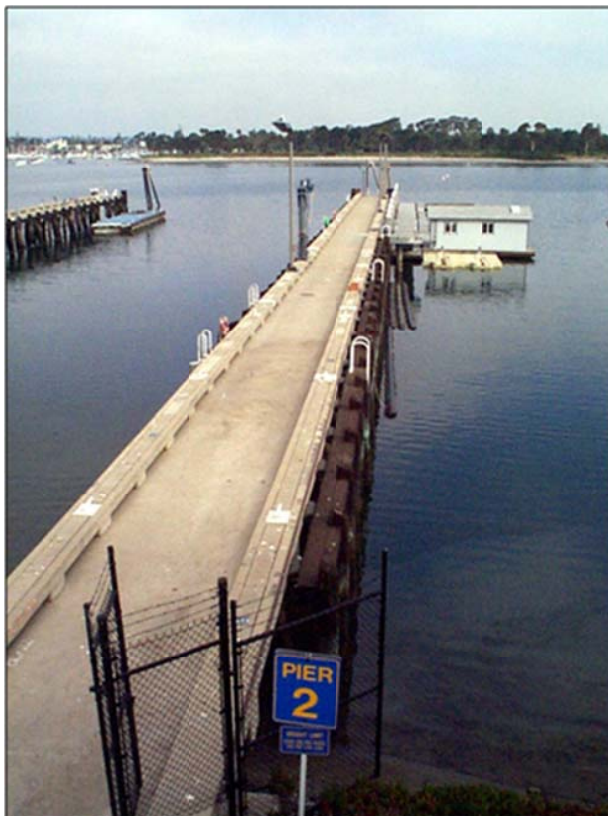
Figure 5-260. Small Craft Pier No.2, NAB Coronado. The pier is representative of 13 piers at NAB. The piers have fender systems for small craft, potable water service, and lighting.
