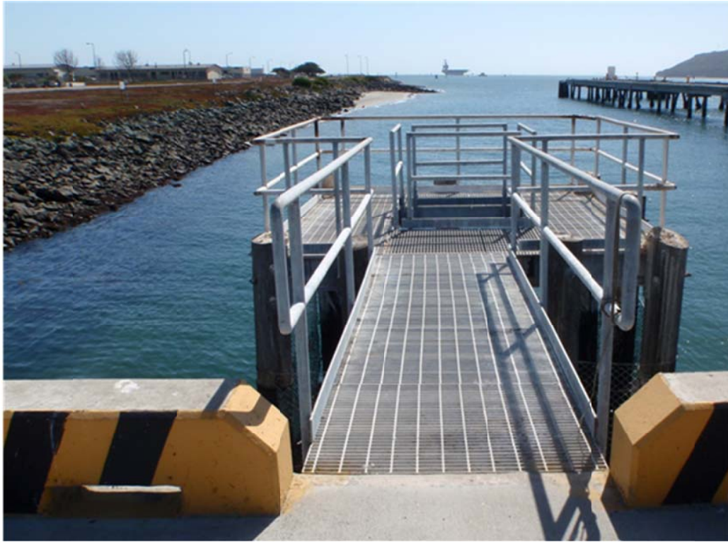
Figure 5-265. Pier Bravo Revetment, NBC.
