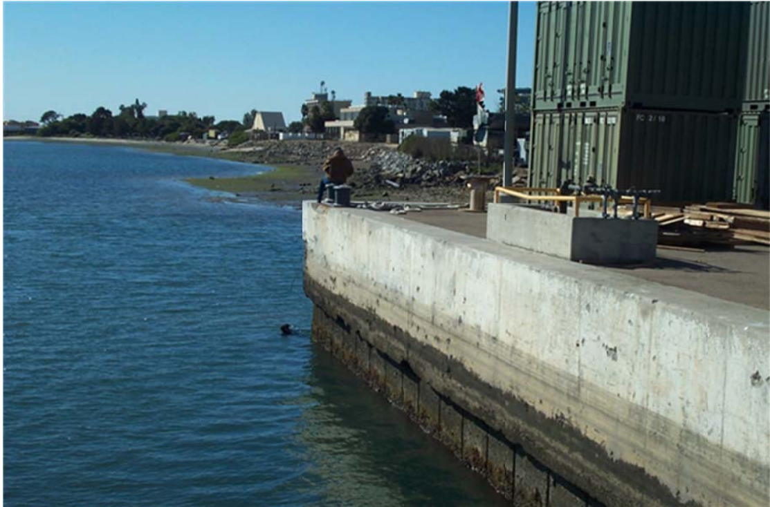
Figure 5-271. Typical Concrete Bulkhead at NAB Coronado.
