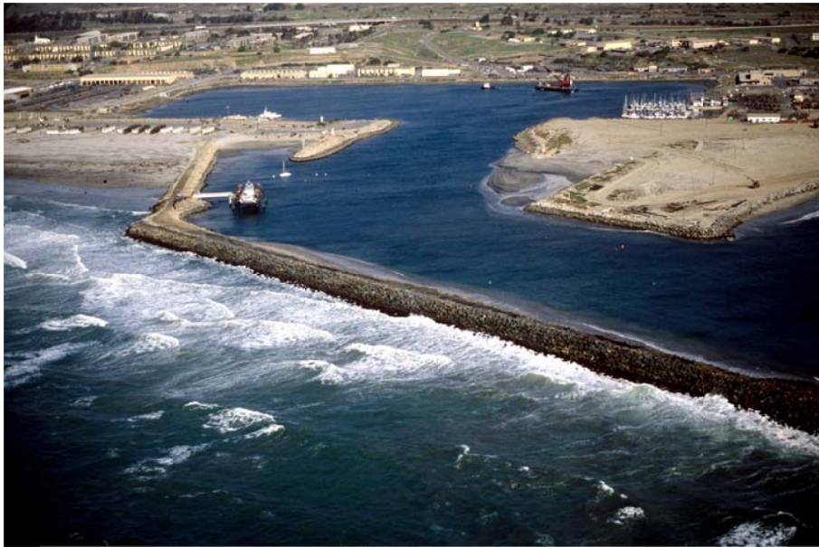
Figure 4-115. Wave breaking on the rubble-mound structure at Oceanside Harbor (California Coastal Records Project Image 8921042; Copyright (C) 2002-2014 Kenneth & Gabrielle Adelman, California Coastal Records Project, www.Californiacoastline.org ).
