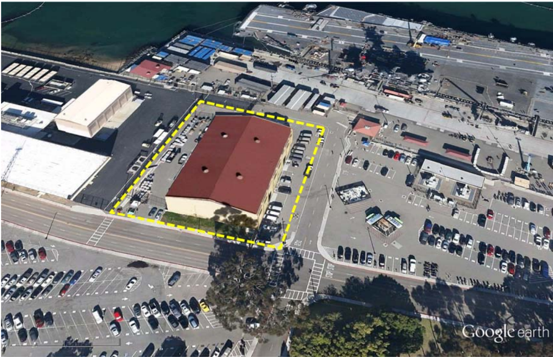
Figure 5-228. A portion of Berth Juliet at NAS Coronado is shown. The yellow outline indicates the CVN Warehouse (Image: Google).
