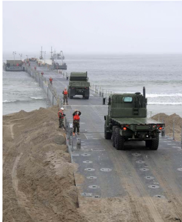
Figure 5-224. Elevated Causeway System training activity. The causeway is anchored to shore, and extends beyond the surf zone (U.S. Navy photo by Mass Communication Specialist 2nd Class Bryan Niegel).
