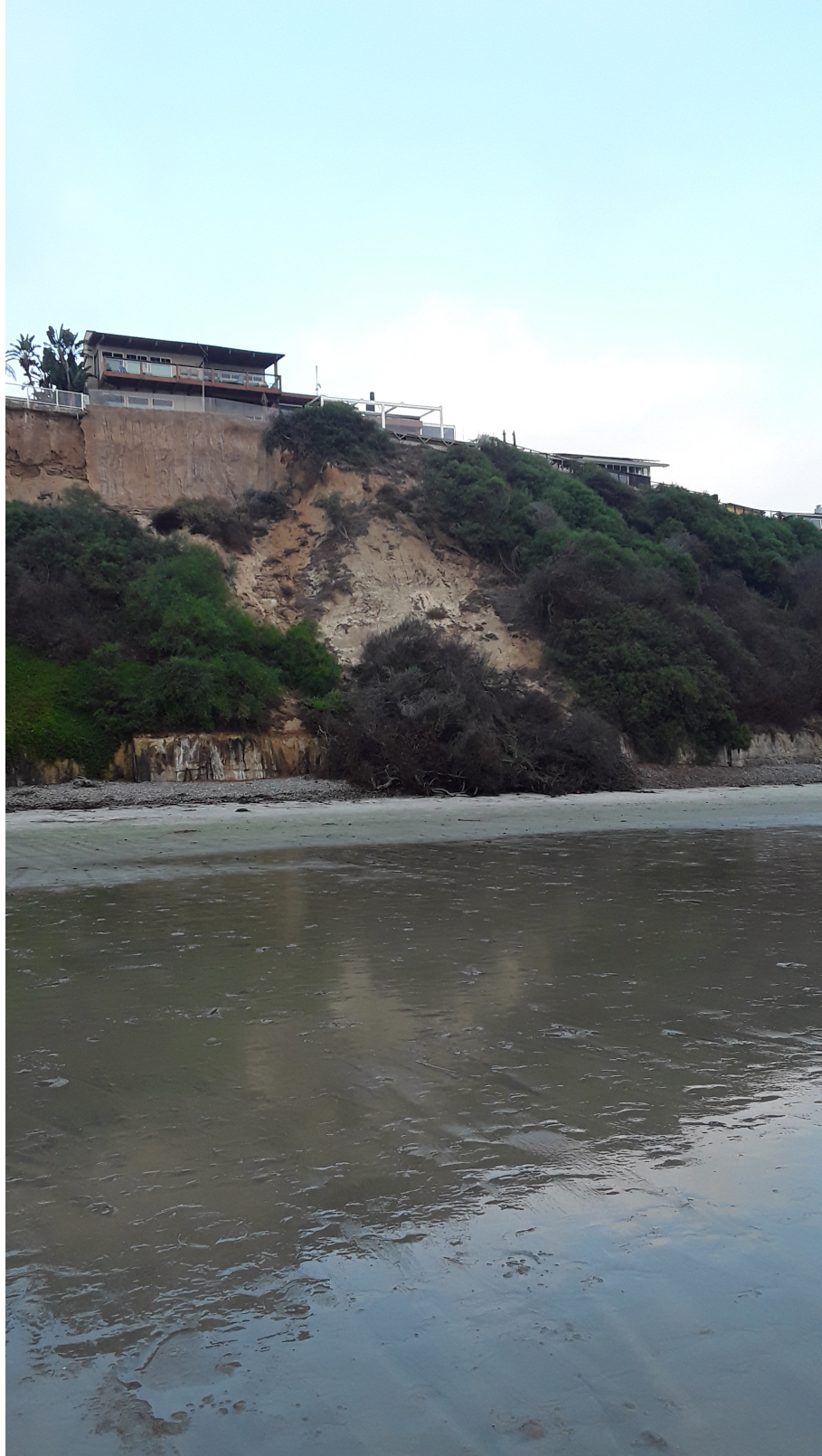
Figure 6: Upper bluff failure example B.
