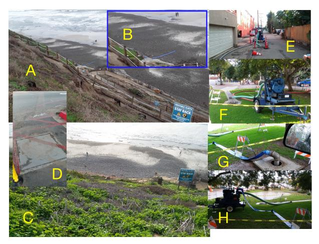
Figure 9: Current pumping approach of moving stormwater onto beach at Beacons Beach.
