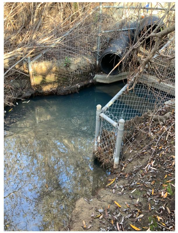
Figure 11: Existing outfall into Batiquitos Lagoon.
