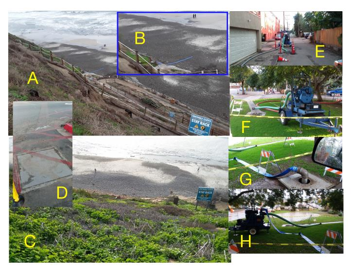
**Figure 6:** Stormwater pumping on to the beach at Beacons. (A) Blue outfall pipe on beach at Beacons. (B) Close-up of pipe. (C) No pipe on beach. (D) Pipe access manhole in Beacons parking lot. (E) Portable, City-operated pump in alley across from Leucadia Park shown flooded in Figure 5. (F) Portable, City-operated pump in Leucadia Park with connections to outfall pipe at Beacons (G), (H).
